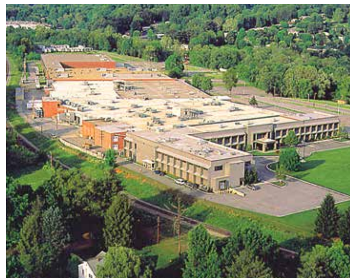
AERUS MANUFACTURING PLANT | BRISTOL, VA
